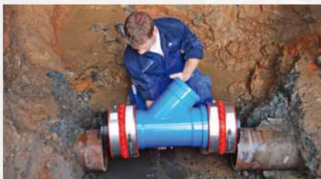
Retrofitting a branch element into an existing vitrified clay pipe
