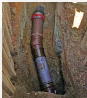
Connecting new pipes
