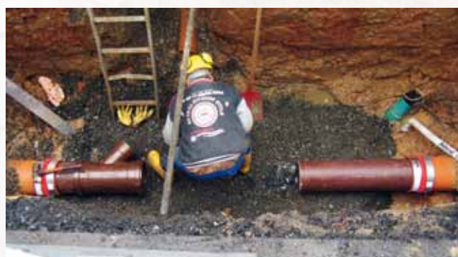
Repairing defective pipes
