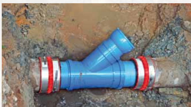
Retrofitting a branch element into an existing vitrified clay pipe
